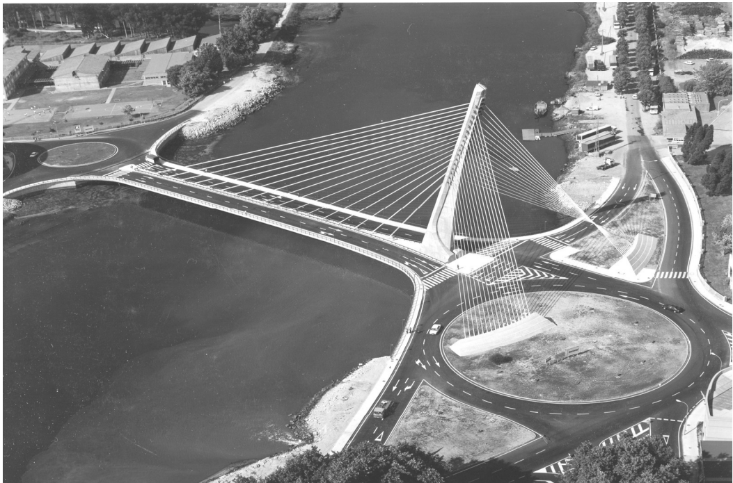
The Puente Sobre El Rio Bridge in Lerez, Spain, is a cable stayed bridge with a main span of 129 m (423 ft) and a prestressed concrete single box deck. (Courtesy Carlos Fernandez Casado S.L.).
